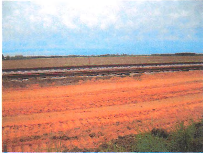
Existing Railway and pipeline orientation
